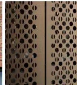
Royal Veterinary College, detail Powder coated aluminium perforated panel
