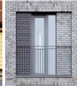
Burridge Gardens, Clapham, detail Gray brick, perforated vent panel, Juliet balcony, soldier course
